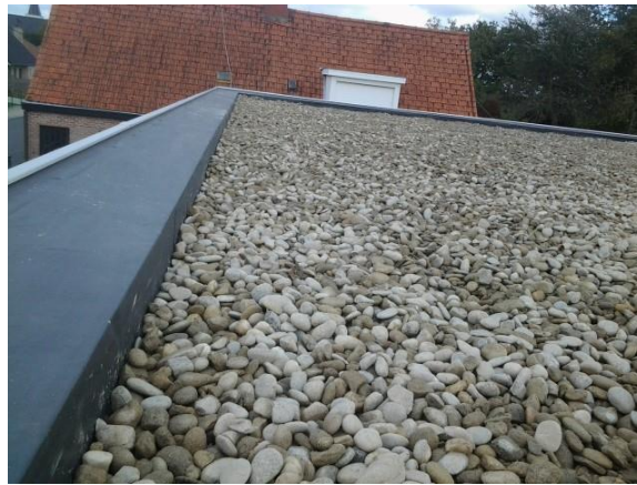
Foto dakplatform in EPDM ter illustratie
